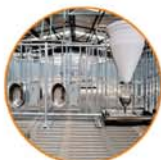
Drinking water system
